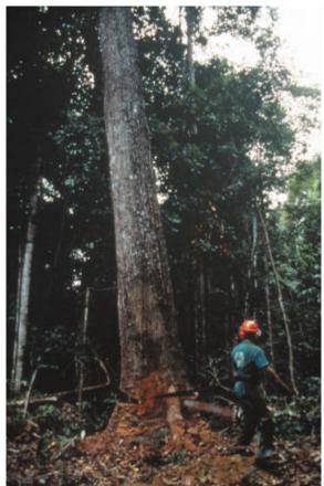
Directional felling is a key step in reducing damage to the residual stand and increasing logger safety.
